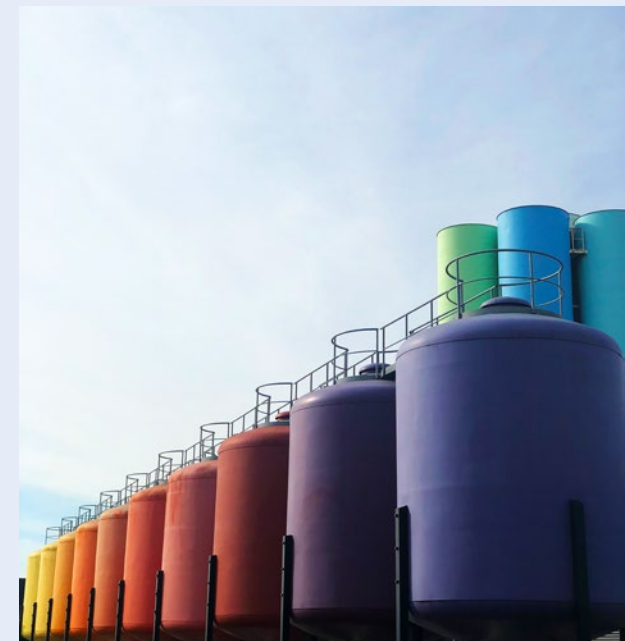
Flügger's factory in Kolding is undergoing a radical modernisation process, one of the objectives of which is to create as clean a production as possible.
